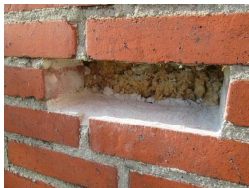
Mineraluldsgranulat i hulmur
